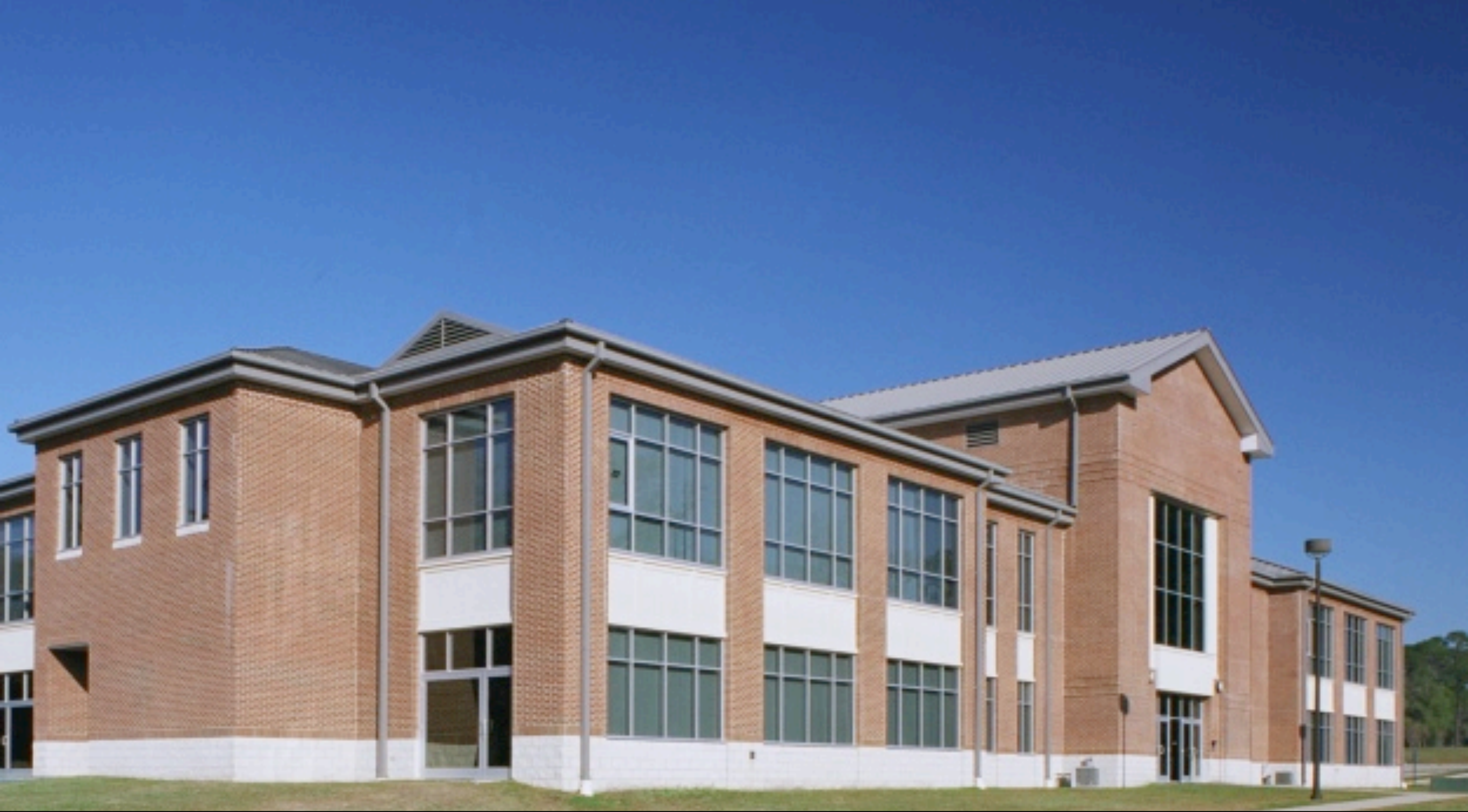
FPSI Classroom Building
